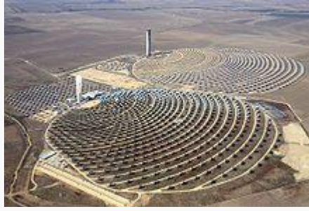
Solar Towers from left: PS10, PS20.
